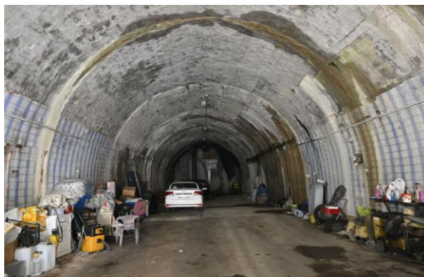
Fig. 2. Portal zone of the tunnel from 1950s (Source: Kaldrma, 2023).
