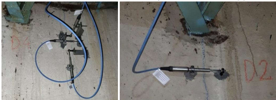
Figure 6. Installed Teledeformeters (Triaxial and Uniaxial)
