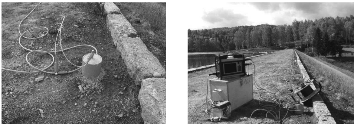
Figure 5. Fixed electrodes on the crown of the filled Vlasina dam for periodic geophysical monitoring (Vasić, 2018) [10].
