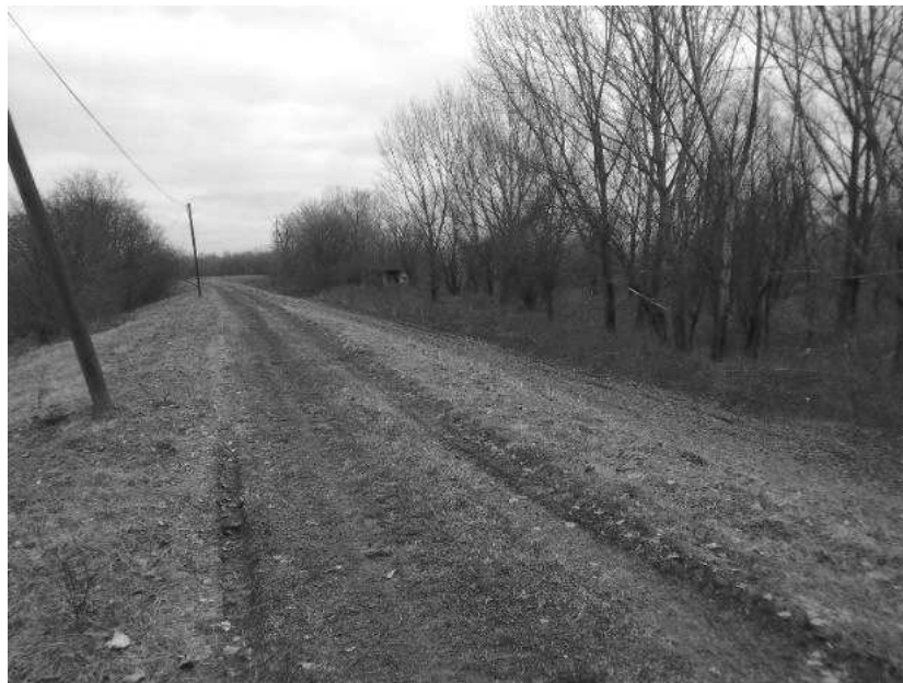
Figure 1. Part of the embankment on the left bank Kolubara which is used as a road for local needs (Kostić, 2019) [2].
