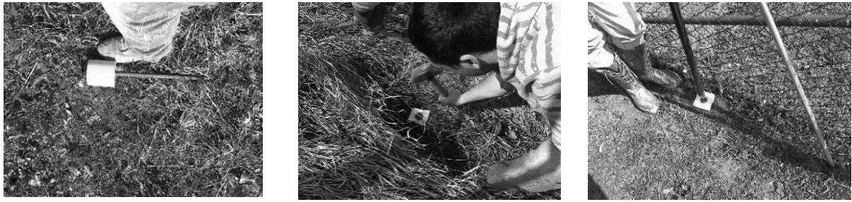
Figure 3. Installation and observation of geodetic landmarks, an example of observation of landslide movement in the hinterland of the Đerdap accumulation (Lazarević, 2017) [8]
