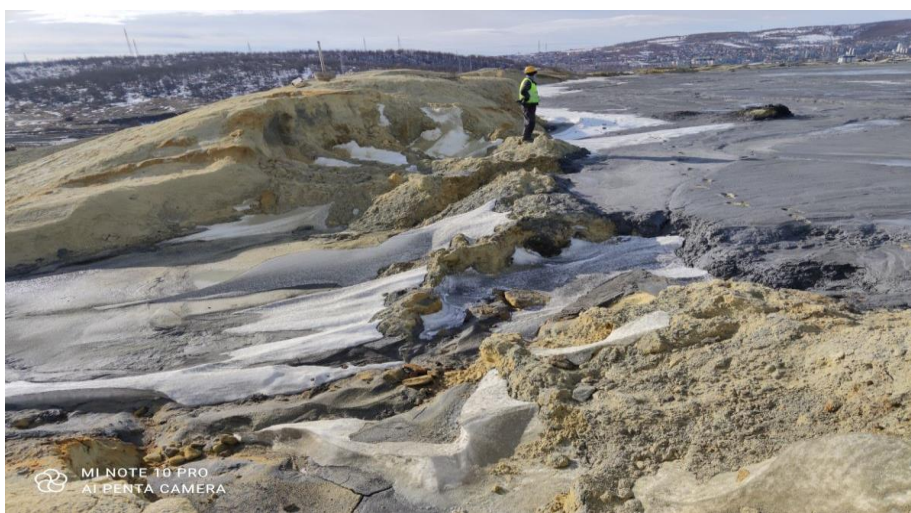
Figure 3 Completely eroded crown of the Dam 2 where the first serious overflows of water and sludge were observed over the crown and downstream slope, January 29, 2021
