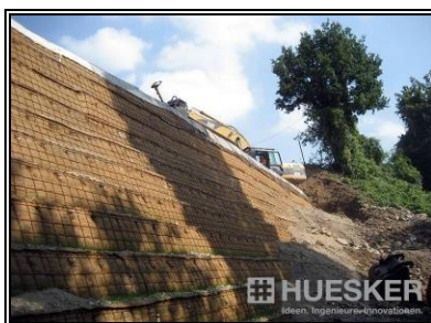
Figure 1 Geogrid of jute, produced Huesker [4]
