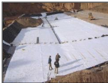
Figure 2 Achieving the erosion stability using geosynthetics [2]
