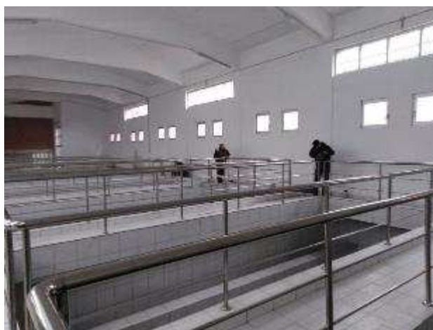
Figure 9: GAC filter facility
