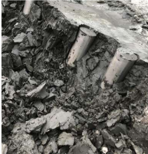
Fig. 9. Frankfurt Clay at Güterplatz, freshly hand-excavated
