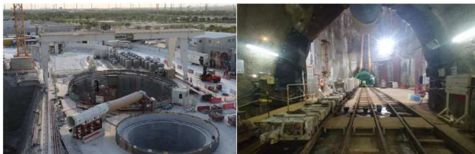
Fig. 5. Photo of the logistics and drop shaft during TBM operations.
