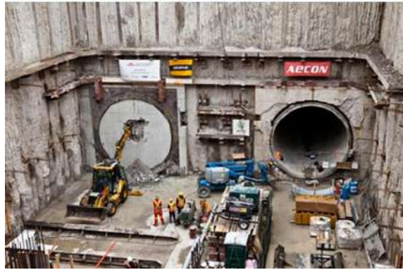
Fig. 3. View of tunnel portal
