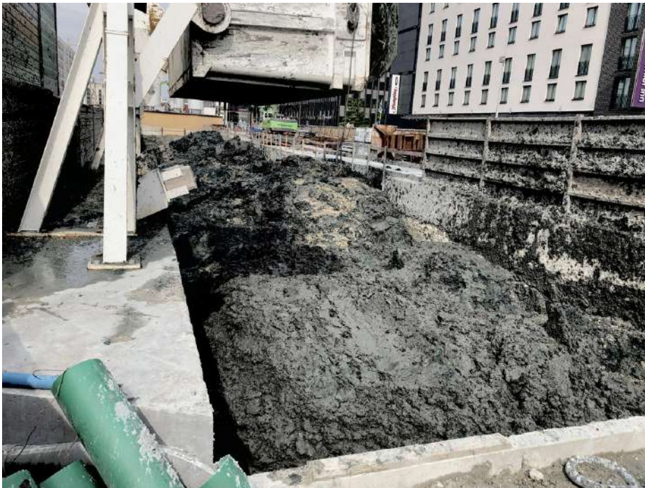
Fig. 12. Conditioned Frankfurt Clay at station surface, June 2020.
