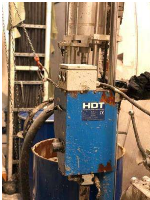
Fig. 15. HDT 200 T press plate pump installed on Herrenknecht gantry.
