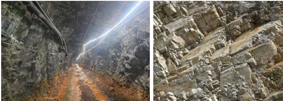
Fig. 4. Very blocky siltstone. Left: fresh siltstone in existing exploration tunnel (3 m wide x 3.5 m high). Right: Slightly weathered siltstone outcrop (approx. 2m high).
