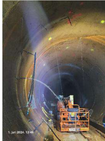
Fig. 15. Installed packers in the right side of the tunnel cross-section at chainage km 7+942.
