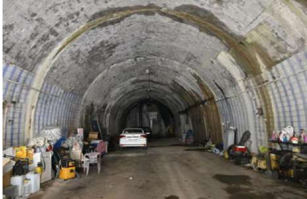
Fig. 2. Portal zone of the tunnel from 1950s (Source: Kaldrma, 2023).
