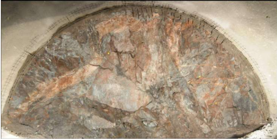
Fig. 2. A typical rock mass condition in the top heading of the repository chambers.
