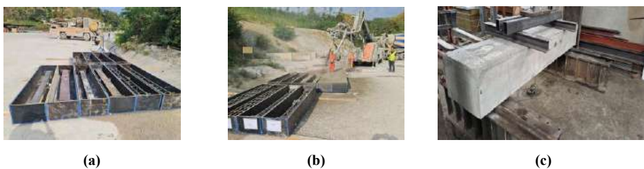
Fig. 3. (a) Lattice girder, steel ribs and reinforcement in the moulds; (b) Shotcrete application; (c) Laboratory testing.
