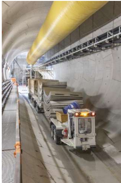
Fig. 3. Project jobsite Grand Paris, photo credit by Eiffage Génie Civil.
