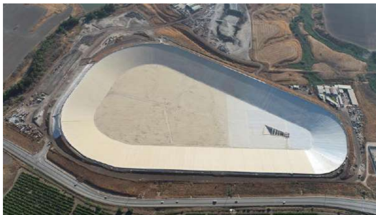
Fig. 1. An aerial photo of the lower reservoir of Kokhav Hayarden pumped storage power plant.
