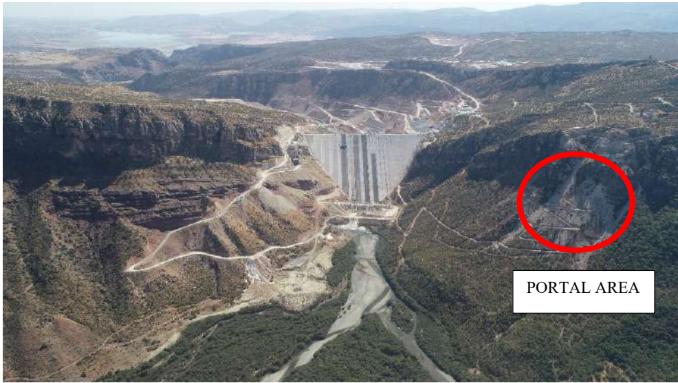
Fig. 2. General view of the portal area.
