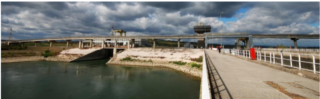
Figure 3. Photo of the additional hydropower plant [3]
