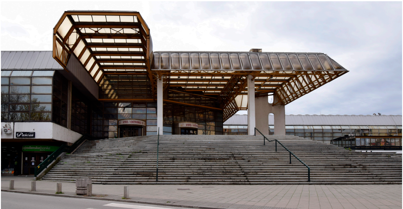
Figure 2. One of Spens' 6 major entrances characterised by large exterior stairs and distinctive polycarbonate and steel roof canopy. Author: Maja Momirov. Copyright 2021 Baza—Spatial Praxis Platform.
