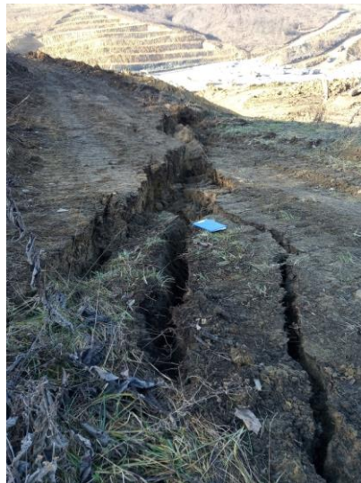
Figure 2.1 Crack in terrain in the immediate vicinity of landslide (December 2020)
