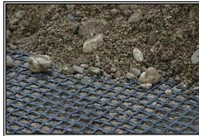
Figure 1. Setting up a geogrid
