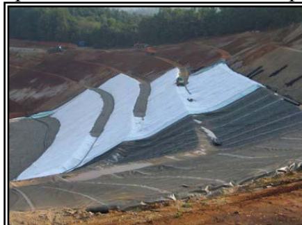
Figure 3. Installation of combined geosynthetic materials
