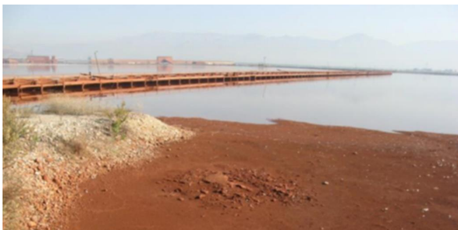
Figure 2. The dam between basins A and B
