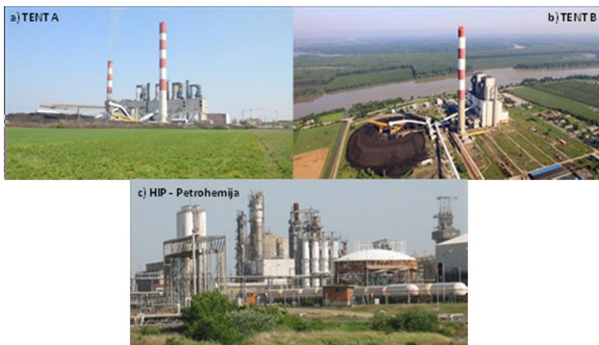
Fig. 1 Republic of Serbia, near Belgrade: Nikola Tesla Thermal Power Plants d.o.o. Obrenovac: Tent A (a) and Tent B (b); industrial-petrochemical complex HIP-Petrohemija a.d. Pančevo (c)
