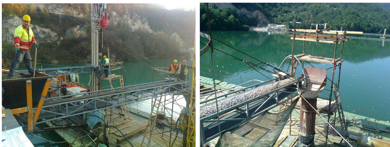
Figure 30. Installation of granular material through boreholes of smaller and larger diameter
