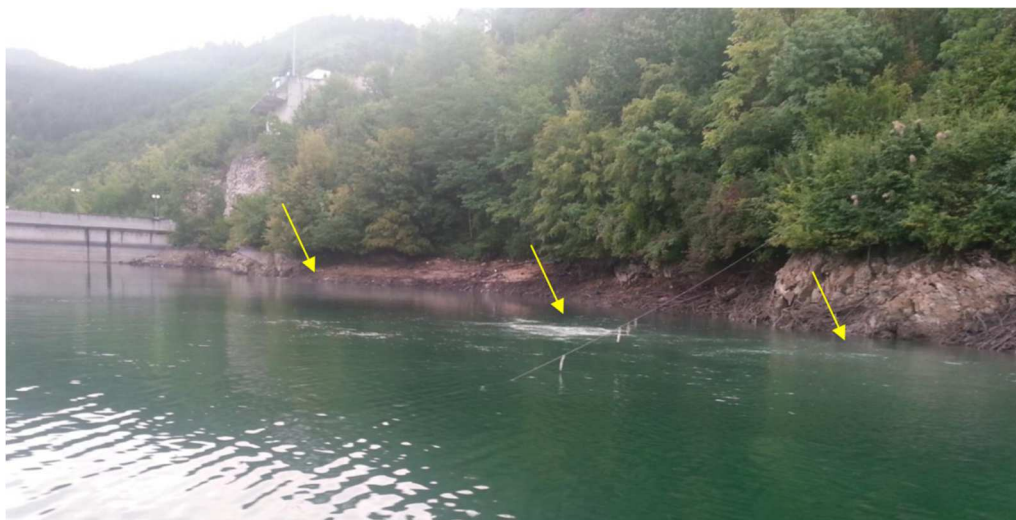
Figure 24. Air outlet in the right flank of the reservoir zone
